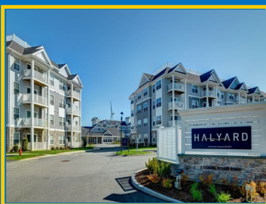
Halyard Apartments School House Road 200 Units / 30 Affordable
